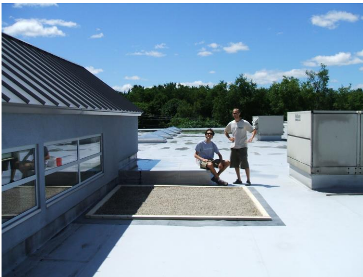
Rounded peastone patch with a frame and landscape fabric, adjacent to a taller section of the building. The wall provides shade but may be too tall.
