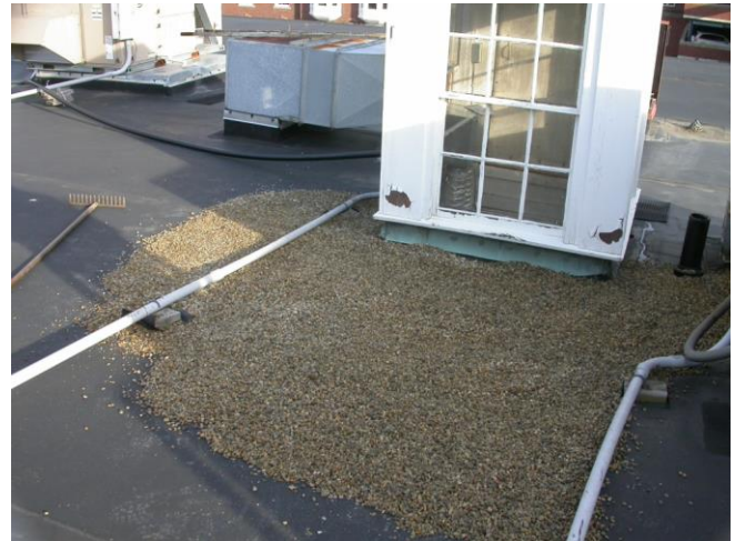
Patch of rounded peastone placed at the center of a roof that had no parapets. Adjacent to cupola for shade.
