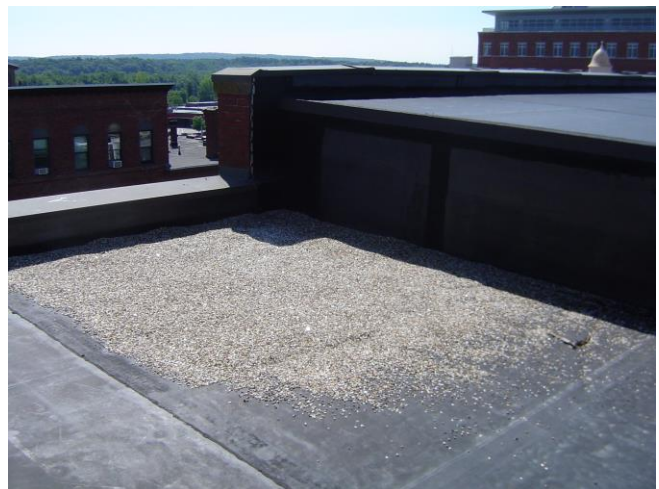
Fracture peastone patch on the southeast corner of one section of a roof. Note the low parapet on one side and the taller wall of the adjacent roof on the other.
