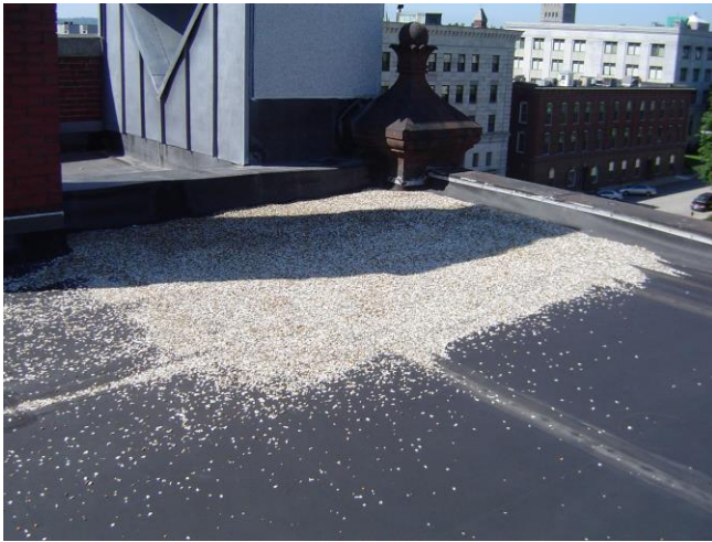
Fracture peastone patch on the southwest corner of a roof with low parapets and adjacent to another roof. Note large structures that may provide too much shade.
