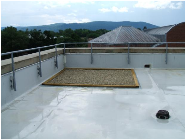
Rounded peastone patch with landscape fabric underneath and a wooden frame.
