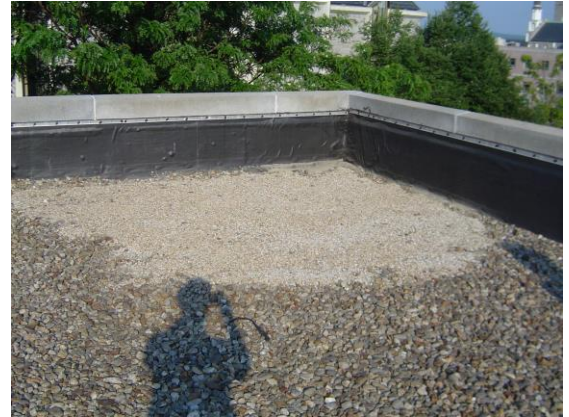
Classic patch location in the southeast corner of a large flat roof. Fractured peastone on top of large stone ballast.
