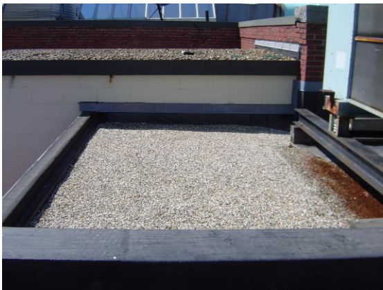
Fractured peastone patch in a small section on the southeast side of a larger roof, but adjacent to another building roof. Note shade from AC unit on right.
