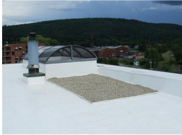
Rounded peastone patch with landscape fabric underneath and a wooden frame.
